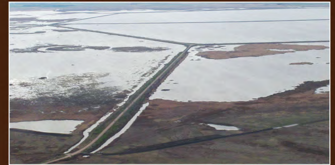
Water control at the bottoms, KDWPT
